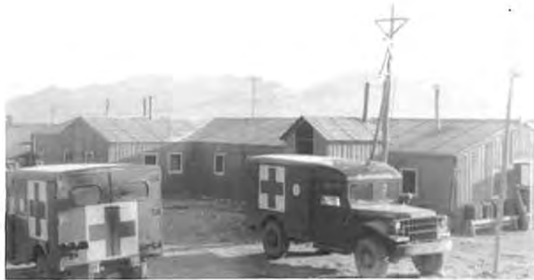
Hospital at 21st Regimental Headquarters
